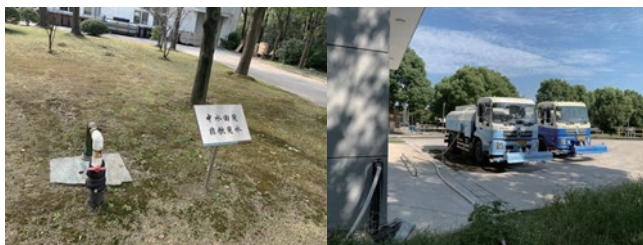
Dazhong Jiading Sewage implement reclaimed water reuse
